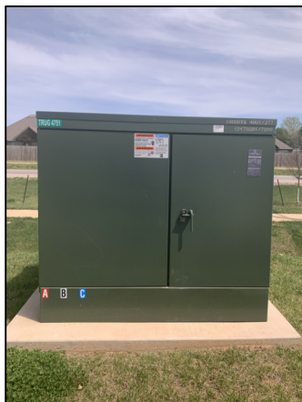
THREE-PHASE PADMOUNT TRANSFORMER
