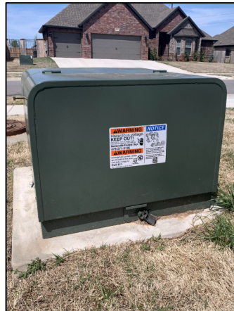
SINGLE-PHASE PADMOUNT TRANSFORMER
