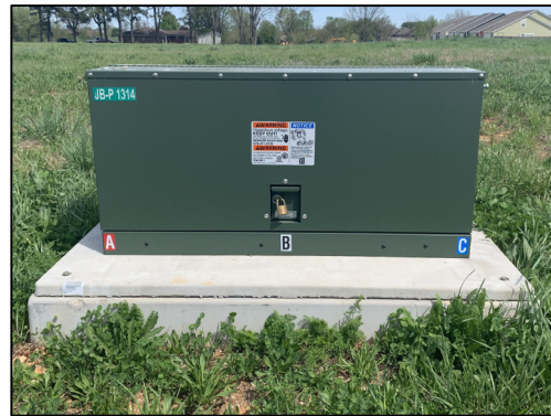
THREE-PHASE PRIMARY JUNCTION BOX
