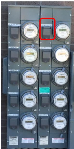
In a multi-unit apartment complex, the main breaker for each unit is typically located in the panel where the meters are installed. Each one should be labeled with the apartment address and unit number. Open the cover to access the breaker. **Contact your apartment complex maintenance department if you need further assistance with accessing the main breaker.**
