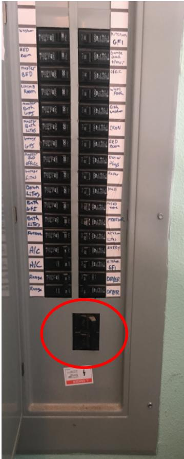
Example of a main breaker located inside the interior breaker panel. It can be located at the top or the bottom of the panel. Some interior panels will have a main panel breaker, but there may still be an overall main breaker for the entire house outside by the meter.
