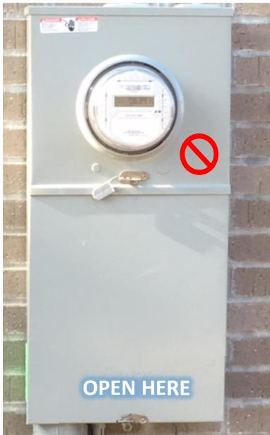
Example of an exterior main breaker location. The main breaker is inside the panel below the meter in this photo. You can open the bottom part of the enclosure, but do not attempt to open the section of the enclosure where the meter is installed.
